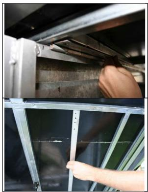
We recommend to fix the piano hinge directly onto the original tent frame.
