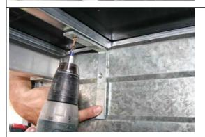
Fix an angle bracket to each of the steel frame sections of the tent from within the trailer. Depending on the size and integrity of brackets used, we recommend 5pcs on each of the 3 walls.
