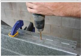
Drill holes in max 10cm distance through the hinge and the side wall of your trailer.
