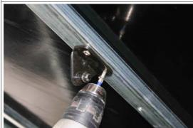
Remove the mounting hinges from the gas struts and fix them with self-drilling screws into the tent frame.
