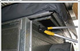
Use a row of rivets with a distance of no more than 10cm to fix the piano hinge directly to the steel frame of the tent.
